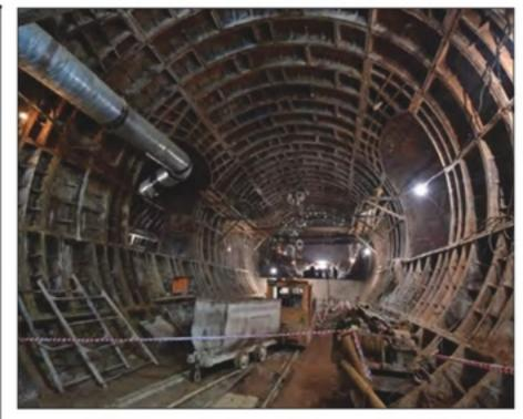
were difficult to implement because of quick soil, an aqueous soil that can liquefy in response to any mechanical impact, such as excavation.
